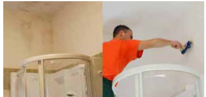
Example of mould proliferation on a wall
