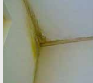
Example of mould proliferation on a wall
