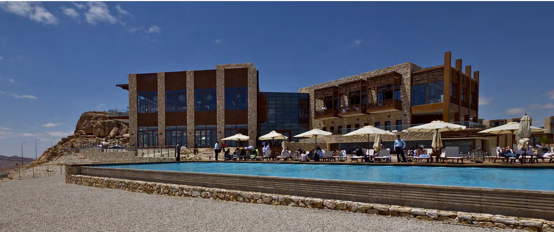
Project: Beresheet Hotel Mitzpe Ramon (Israel) Client: Isrotel Architect: Feigin Architects
