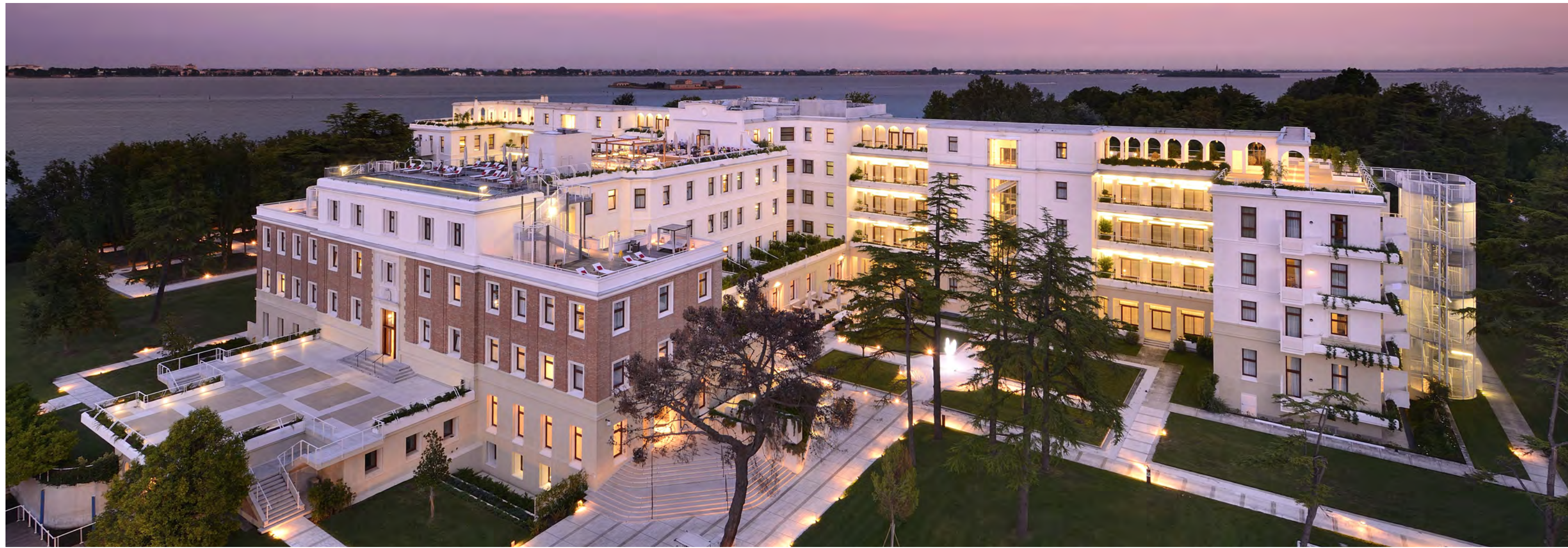
Project: JW Marriott Resort & SPA Isola delle Rose Laguna di San Marco (Venezia – Italy) Client: Sacca Sessola srl Architect: MTLC arch. Luca Colombo
